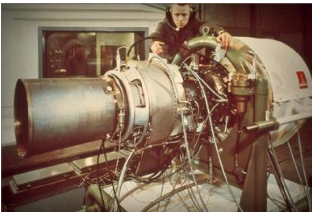
1969 – T53 turbo shaft engine on the test bed
